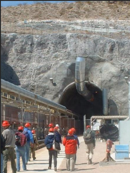
Yucca Mountain tunnel entrance
